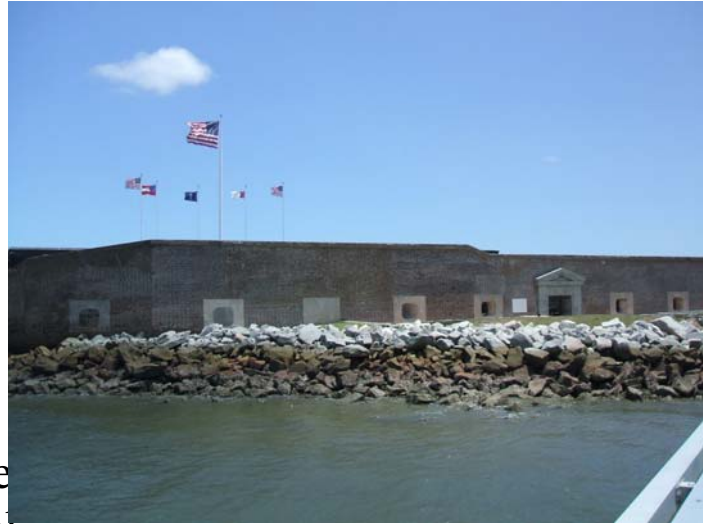
Ft. Sumpter approach today from Charleston
